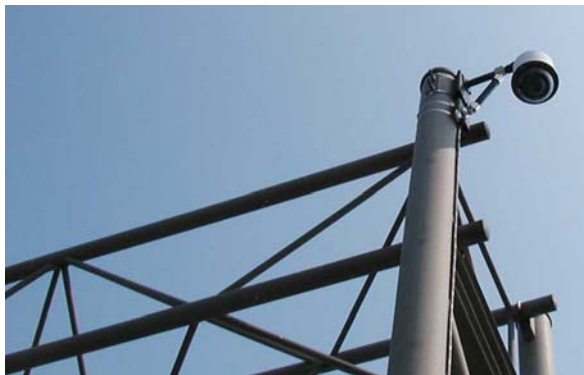
Figure 6-57 Portable CCTV Camera for Freeway Surveillance
