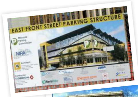
Photos of the Park Place Garage During Construction
