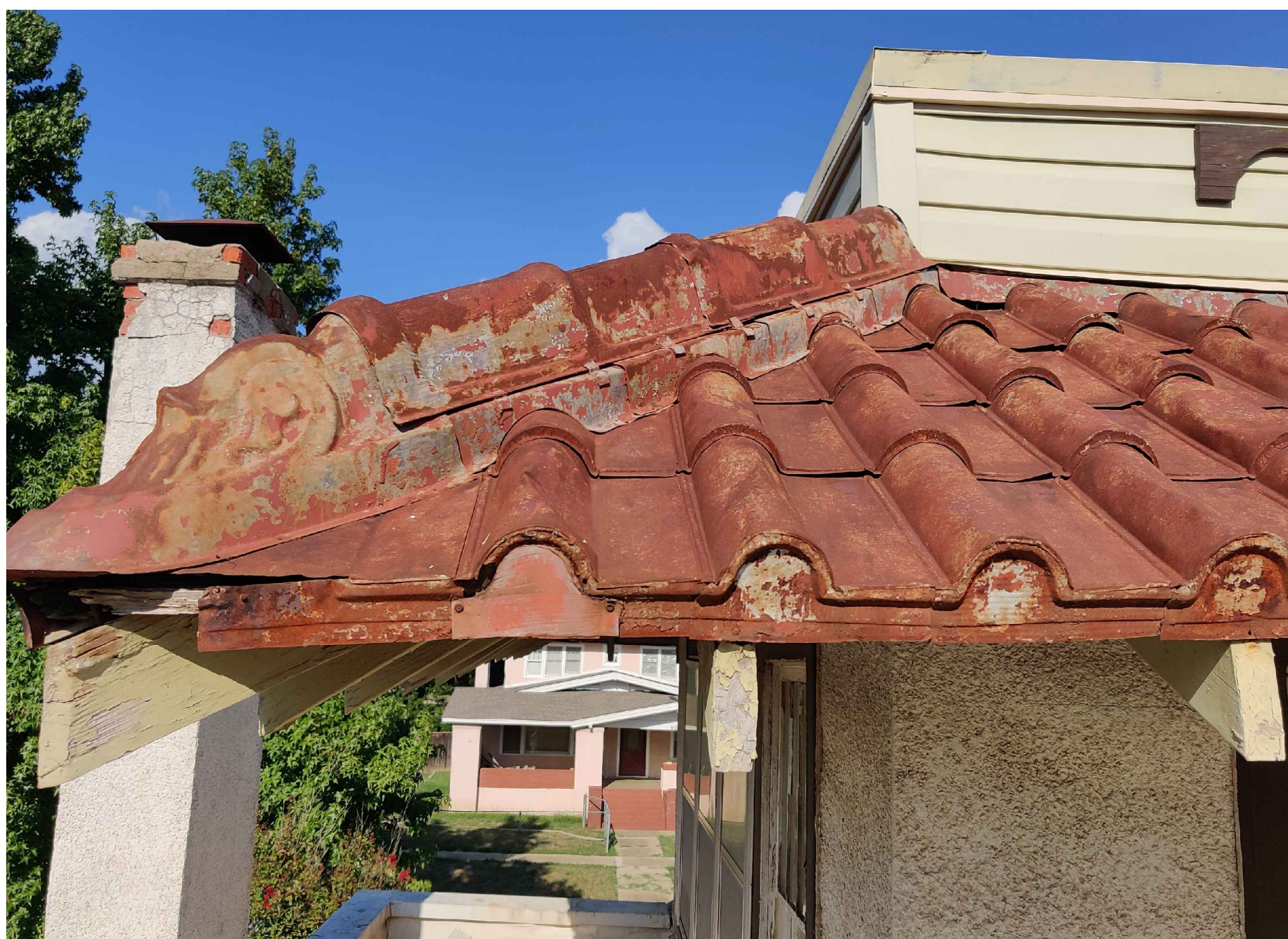
PHOTO- TYPICAL METAL ROOF PANEL AND HIP TRIM
