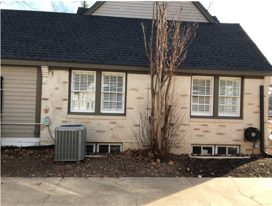
West side of house near front
