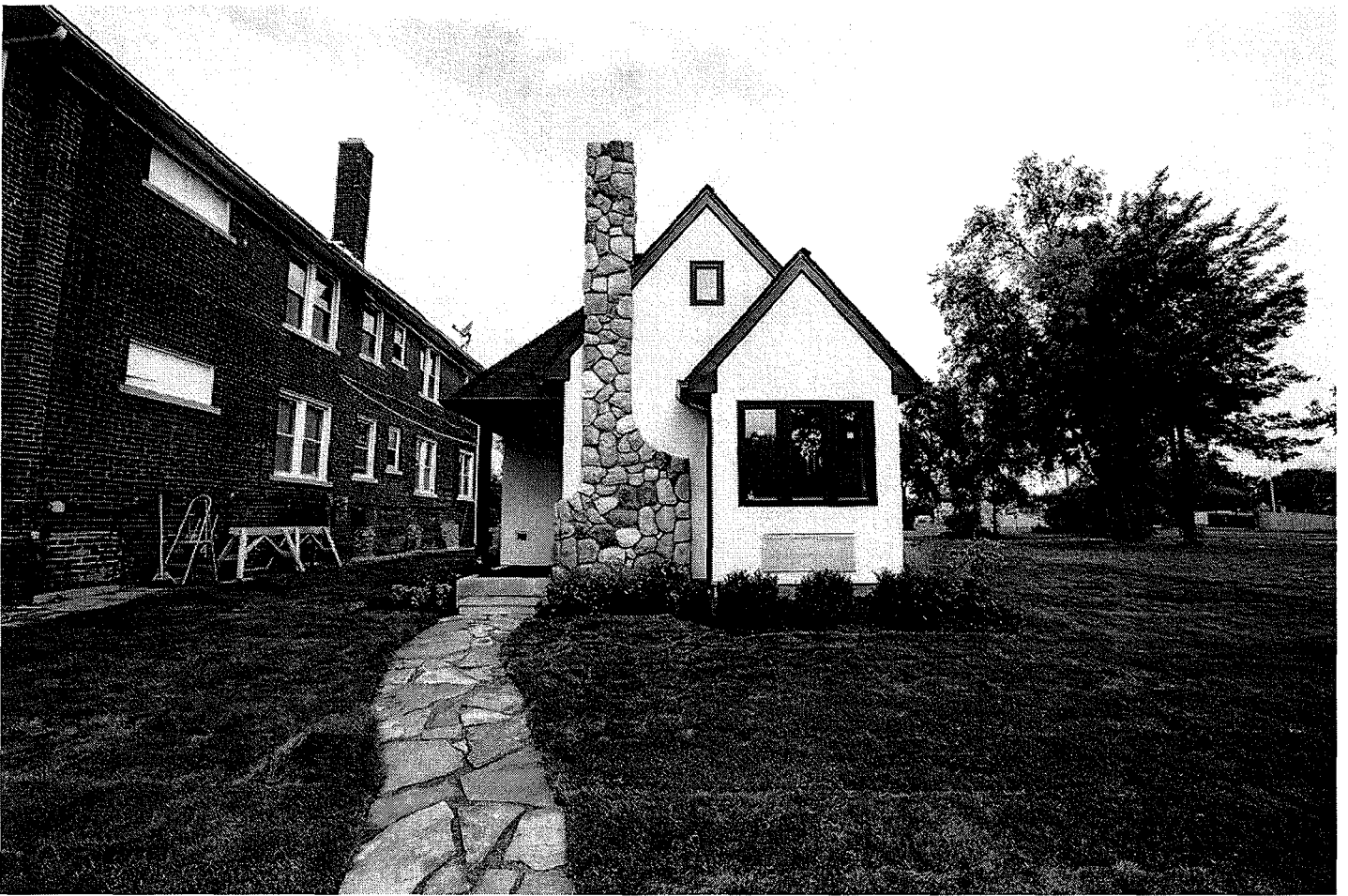
This 300-square-foot home in Detroit is part of an in-development community by Cass Community Social Services for low-income residents. | Michelle and Chris Gerard
