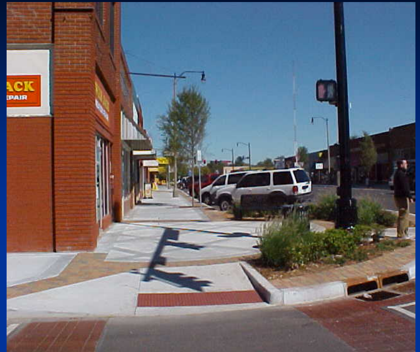
The "look" after improvements
