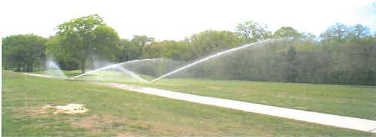
Figure 9 – City of Norman Treated Effluent Application
