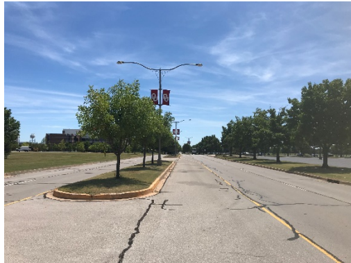
Jenkins Avenue LED Roadway Lighting
