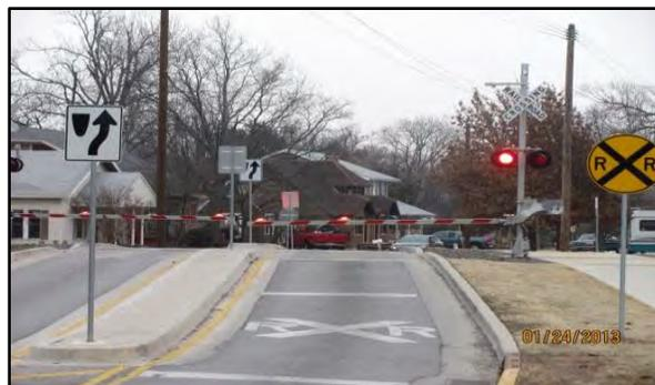
**Automatic gates are provided for frequent crossings by BNSF’s Mid-Con rail line**
