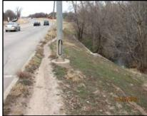
Examples of missing segments and well-worn paths are considered gaps within the existing sidewalk system
