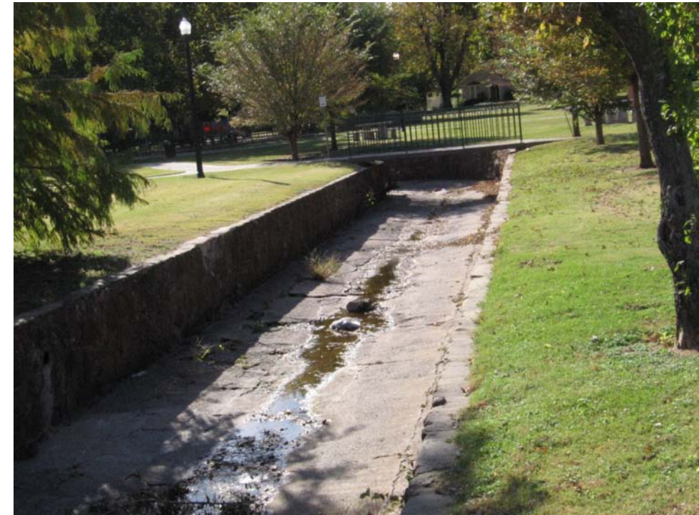
WPA channel downstream of Flood Avenue – Imhoff Creek
