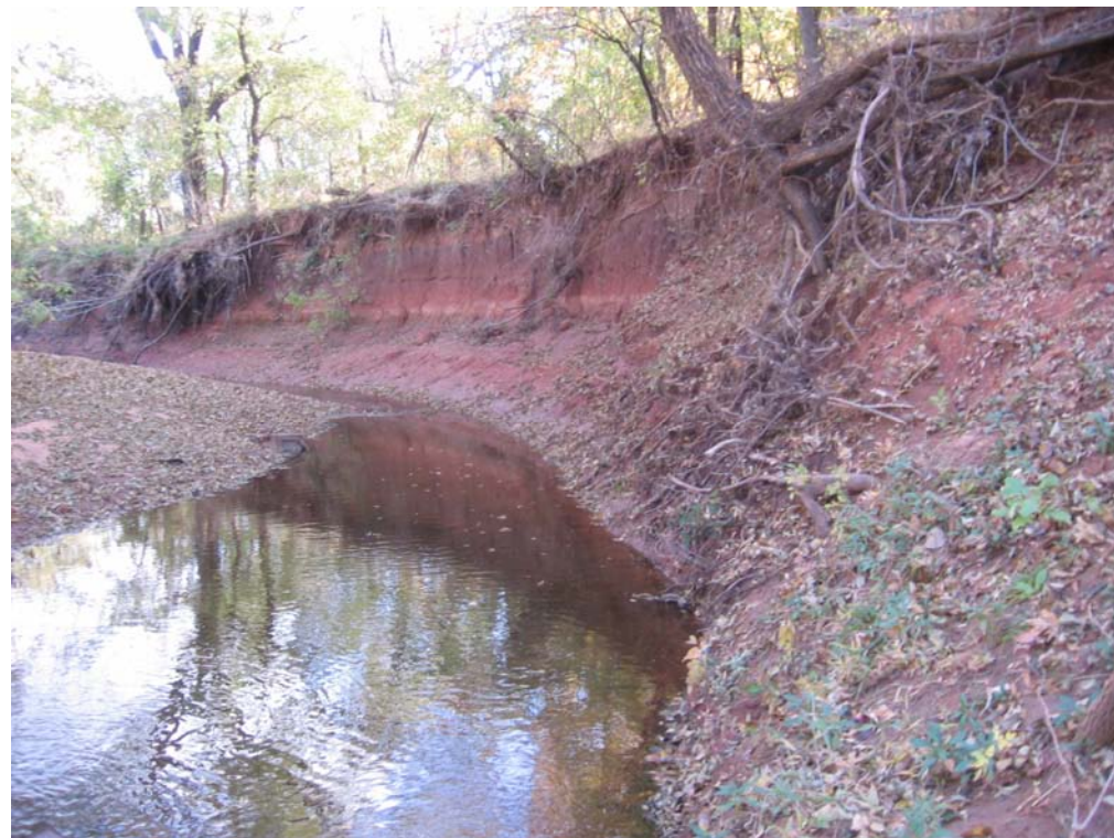
Eroding stream bank upstream of 12th Avenue NW – Little River
