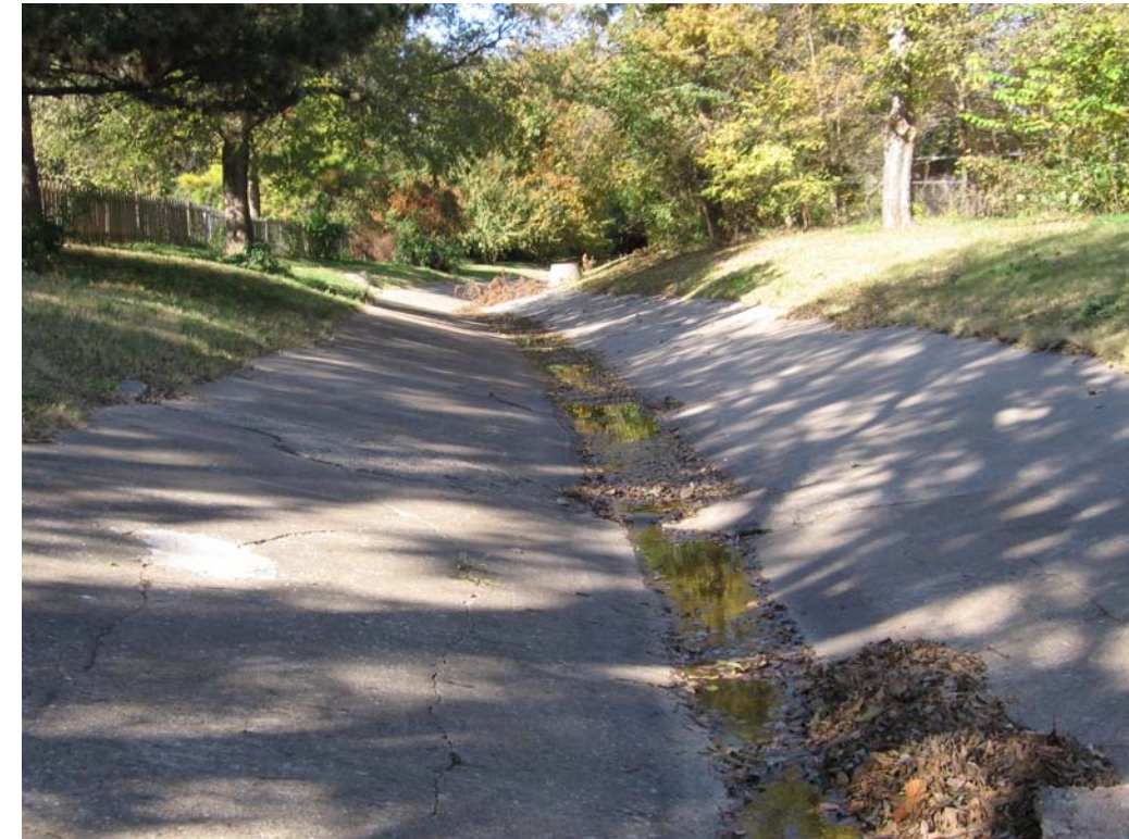
Concrete-lined channel upstream of Lindsey Street – Imhoff Creek
