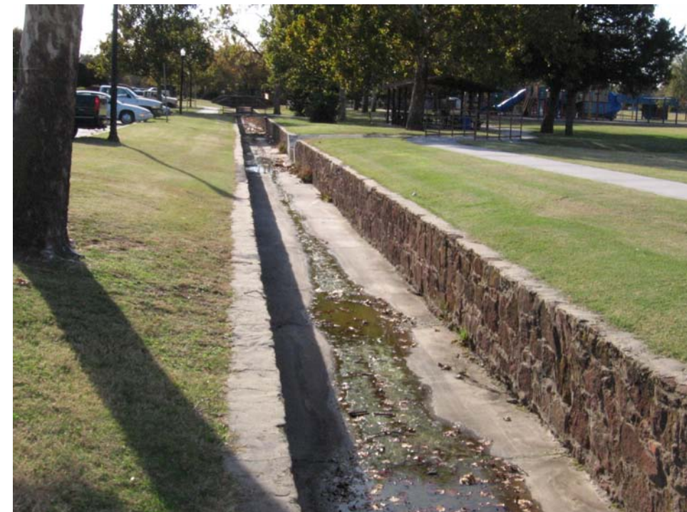
WPA channel in Andrews Park – Imhoff Creek
