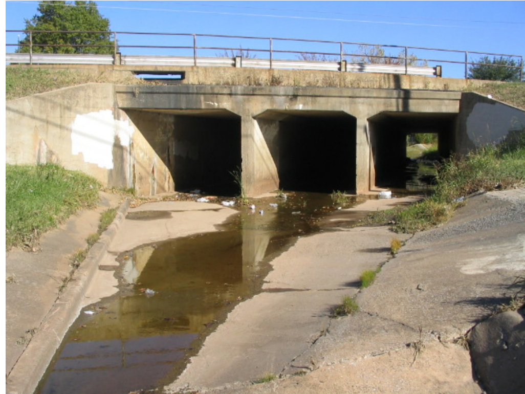
Culvert outlet downstream of Main Street – Merkle Creek
