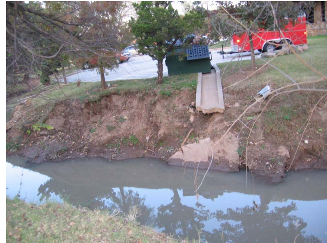
Eroding stream and drainage outfall downstream of 36th Street NW – Brookhaven Creek
