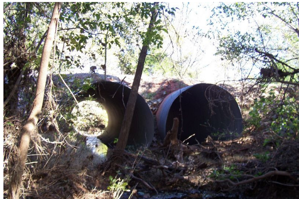
Culverts upstream of 48th Avenue SE – Dave Blue Creek
