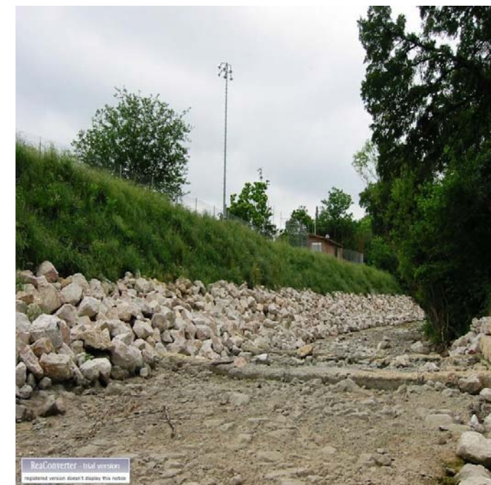
Stream stabilized with MSE design; wastewater infrastructure protected
