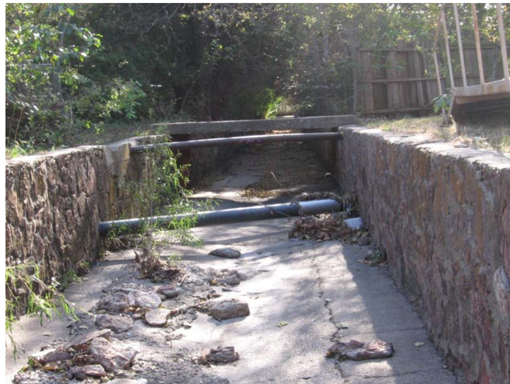
WPA channel downstream of Daws Street – Imhoff Creek
