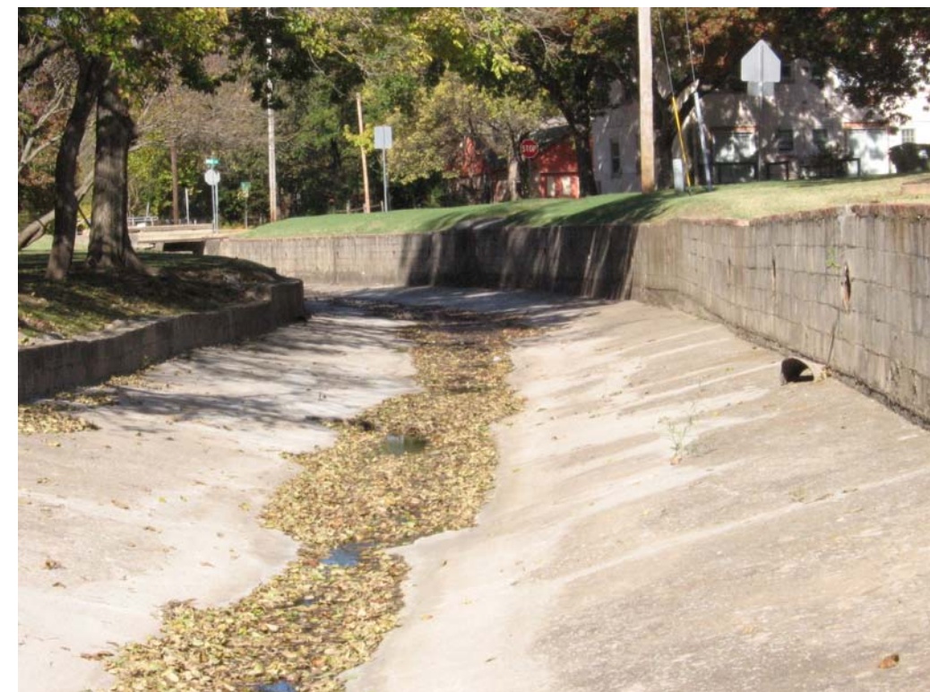
Concrete lining and vertical walls downstream of Boyd Street – Imhoff Creek
