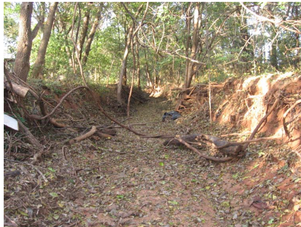
Stream erosion downstream of Sequoyah Trail – Woodcrest Creek
