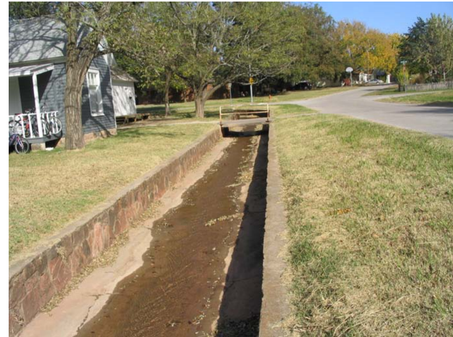
WPA Channel downstream of Carter Avenue – Bishop Creek
