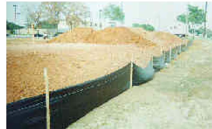
Construction erosion protection with silt fence
