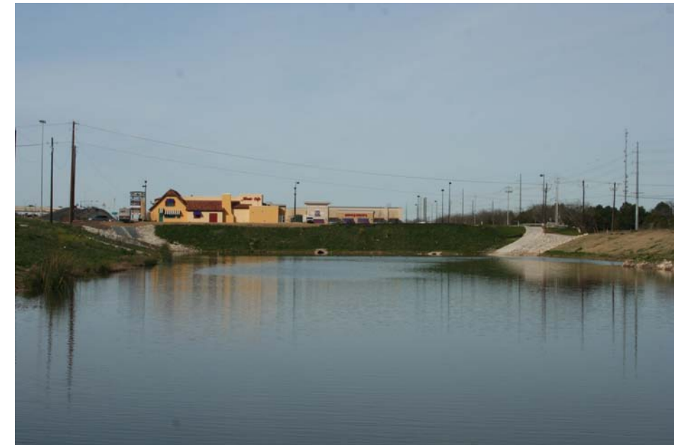
Combination water quality and flood control facility
