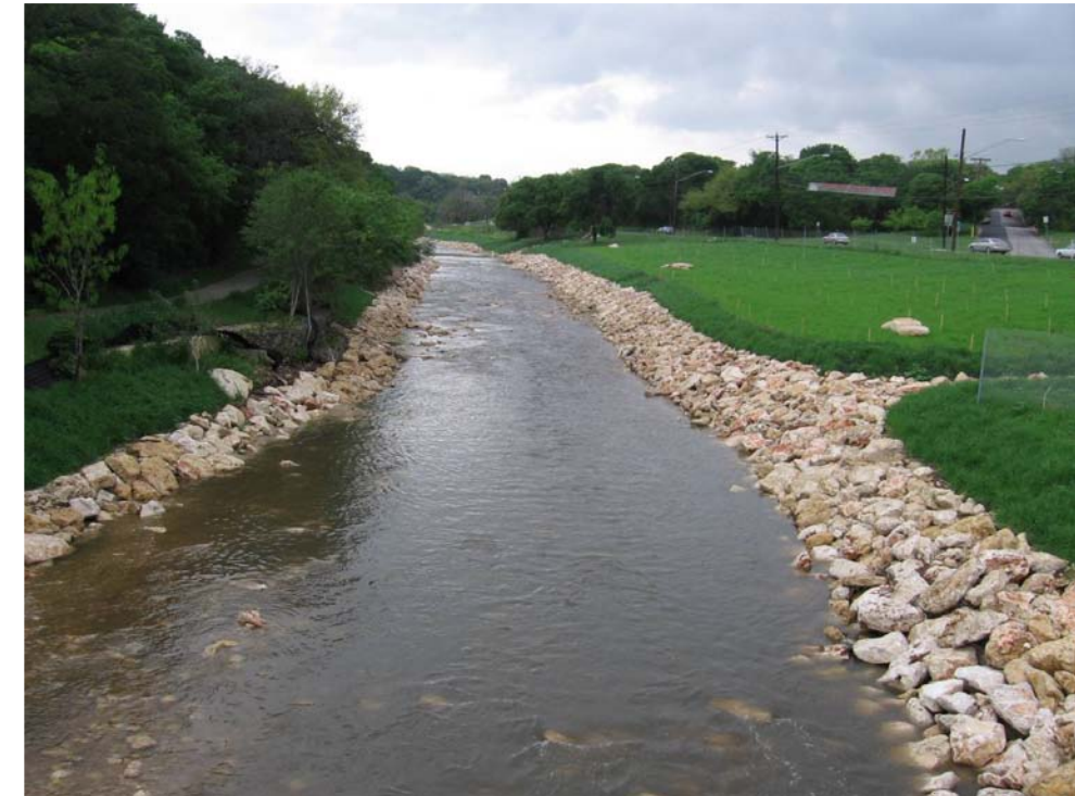
Stabilization using rock riprap
