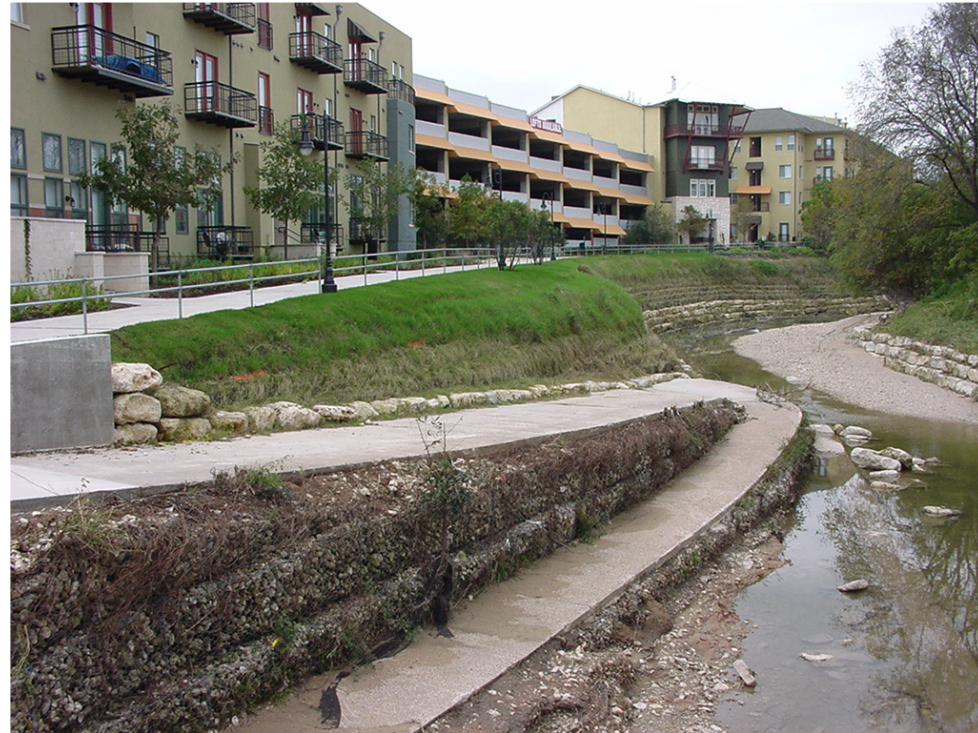
MSE stabilization with gabions and ledge rock in dense urban setting
