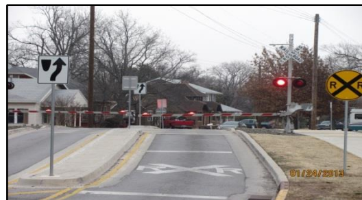
Automatic gates are provided for frequent crossings by BNSF's Mid-Con rail line
