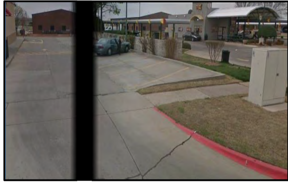
Corner 4 No Ramp (4z)
