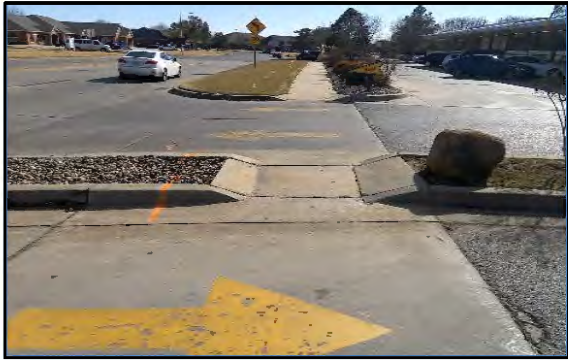
Ramp West F
