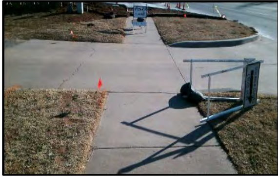
Corner 2 No Ramp (2z)
