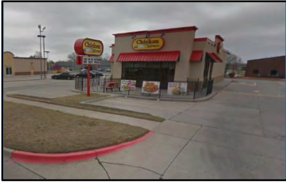
Corner 3 No Ramp (3z)
