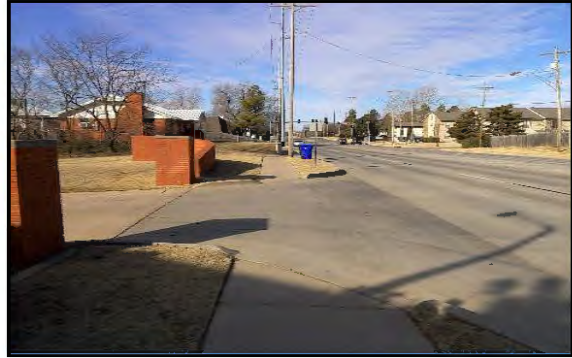
Corner 4 No Ramp (4z)
