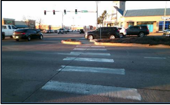
Ramp East F
