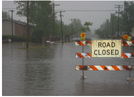
No. 1 Storm Water Problem in Norman (“Lake McGee”)
