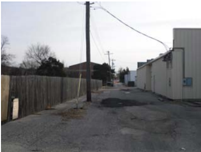
This asphalt alley east of Porter Avenue has been often patched. Board fence separates the alley from adjacent back yards.
