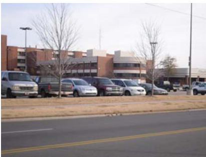
From a neighborhood perspective, Norman Region Hospital is both an asset and a liability.
