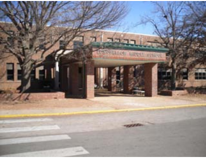
Longfellow Middle School can be a community gathering place as well as a school.
