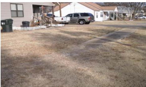
Sidewalk segments along Hughbert Street across from Jefferson School have virtually disappeared under creeping sod.
