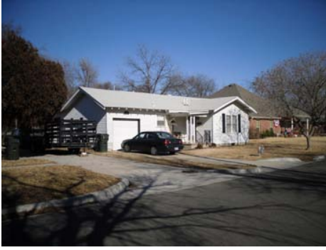
Modest sized, single-family houses are the dominant land use pattern in First Courthouse neighborhood.
