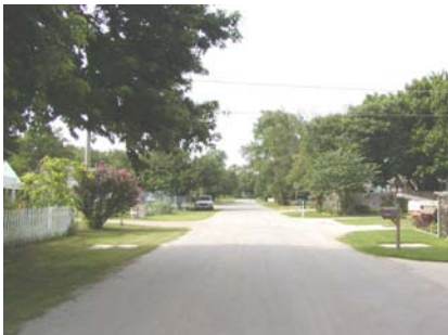
Along some streets in the northern parts of the neighborhood, there are no drainage structures in place.
