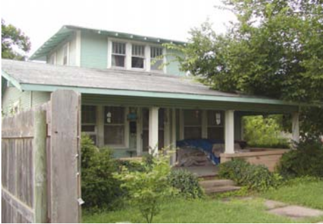
Old Silk Stocking is a comfortable residential neighborhood defined by trees, sidewalks and houses with front porches.
