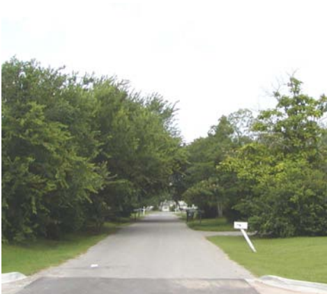
Lack of formal infrastructure and poor drainage along some streets creates problems during heavy rains.
