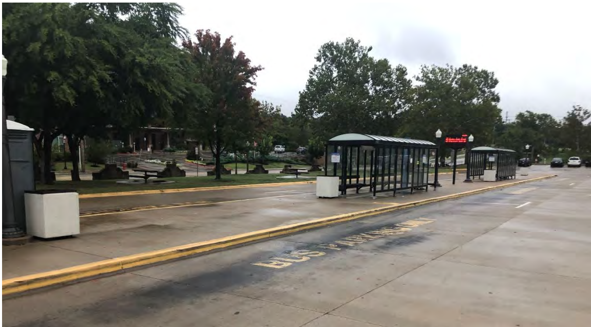
Figure 4-1 Brooks Street Transfer Station
