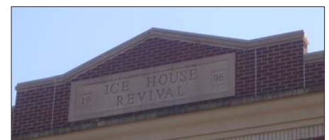
Masonry parapet sign
