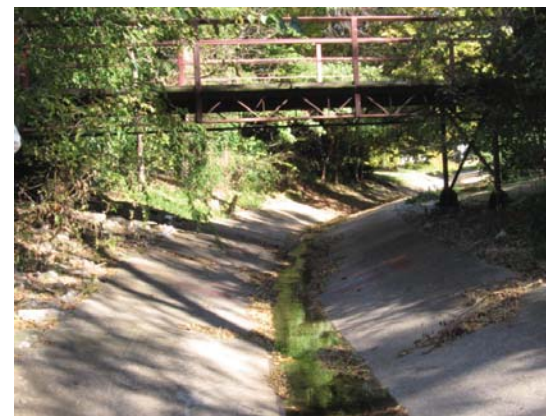
Older creek crossing on the Imhoff Creek
