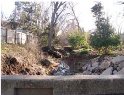
Eroded banks indicate that high volumes of water occasionally flow through this segment of Bishop Creek
