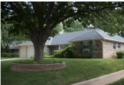
An expectation that property will be well-maintained is a cornerstone of a high quality of life in any neighborhood.
