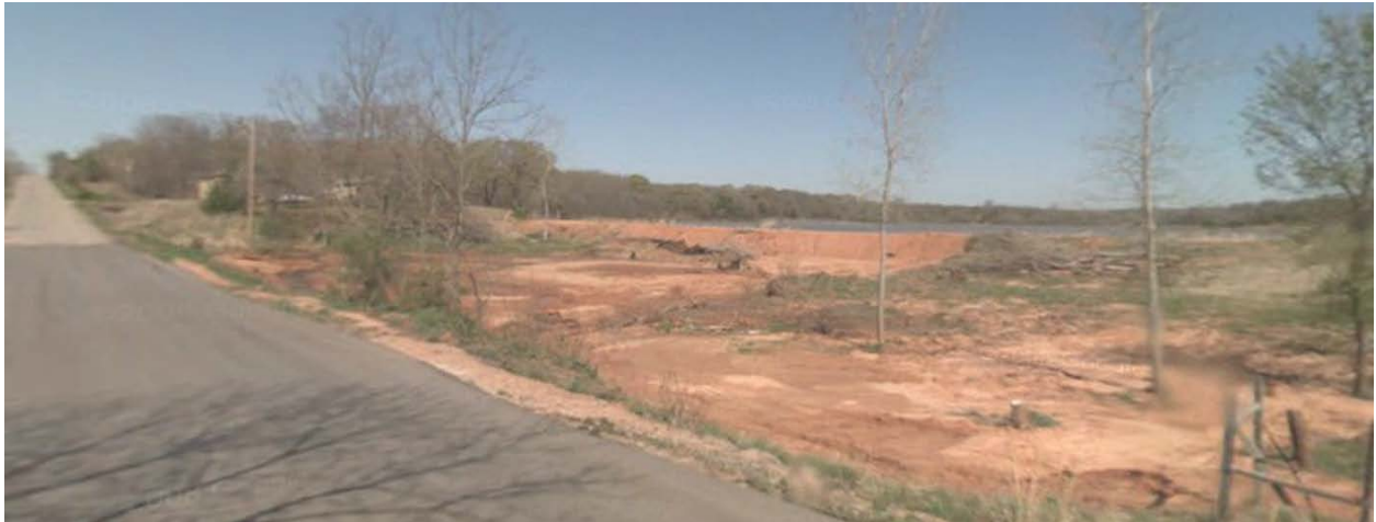
Looking northwest from Reynolds Road to the Reynolds Lake Dam.
