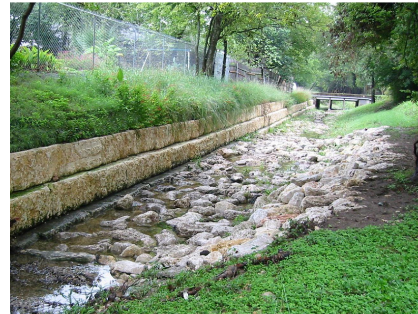
Stream conveyance improvements and stabilization in urban setting
