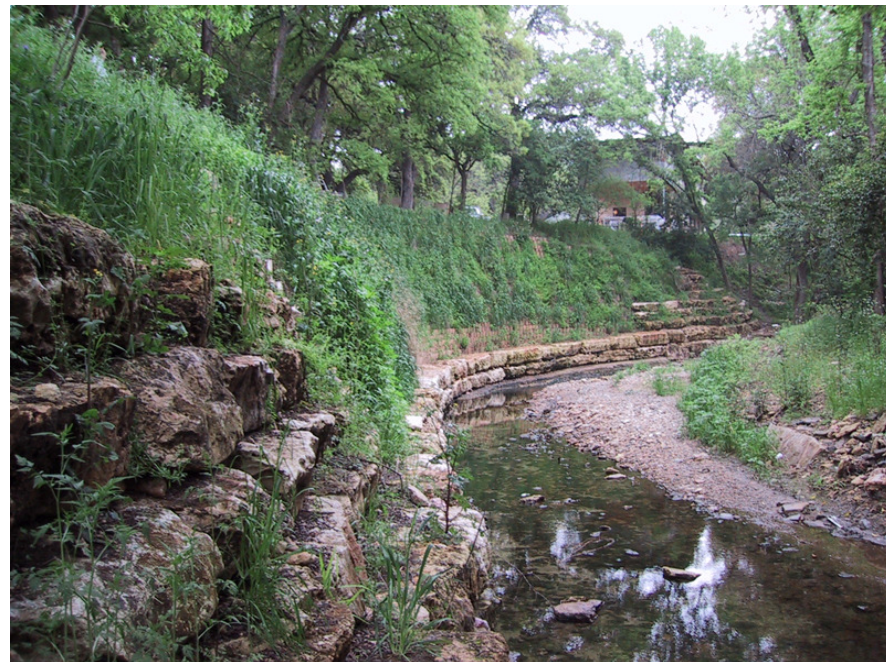
Stream protection along steep bank
