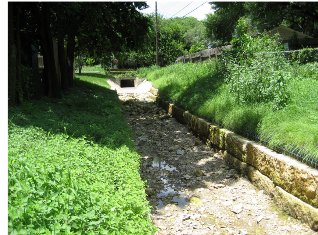
Stable stream section using low-flow channel and vegetated side slopes
